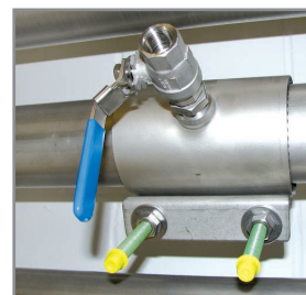
B Spot drilling collars
